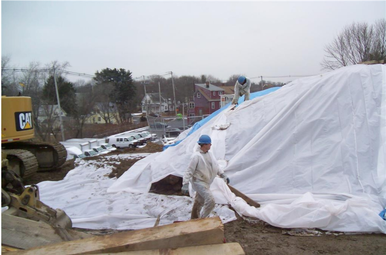
Stockpiled contaminated soil awaiting removal at the Route 35 (High Street) interchange.
